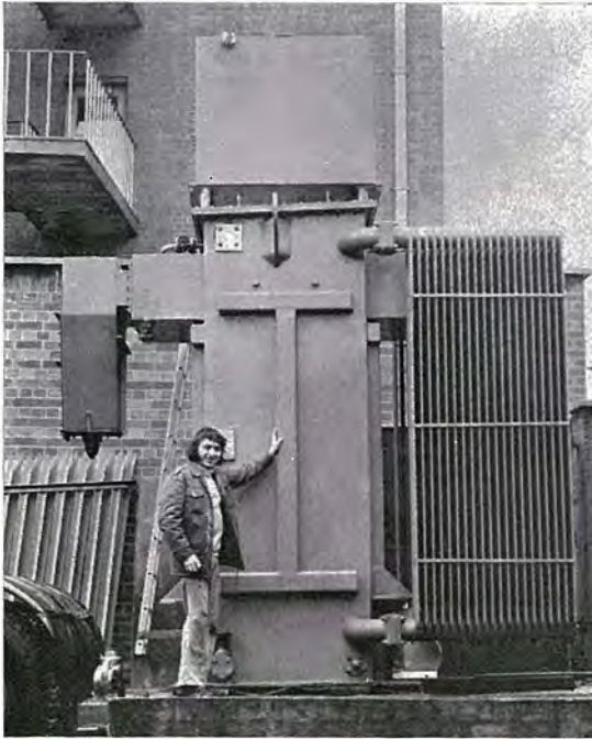
The radiator and conservator on this huge transformer had to be 'craned' into place before the whole unit was lifted into the substation.
